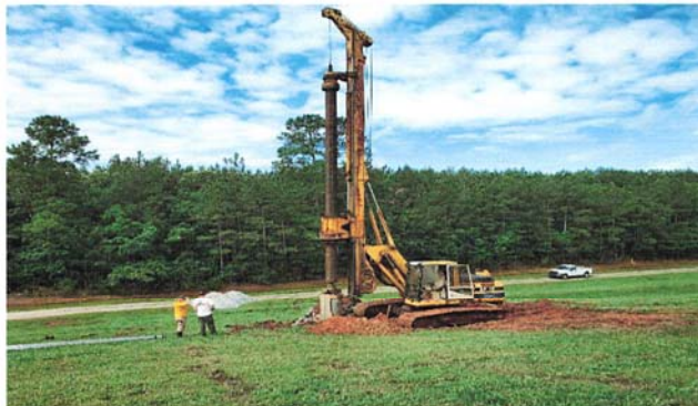
Installation Photo – Vent Wells (June 2020)
