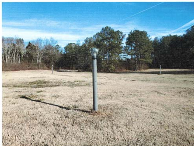
Current Photo – Vent Wells (2021)
